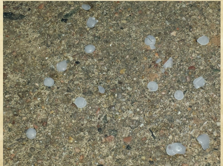
Deicing salt on a concrete sidewalk.
